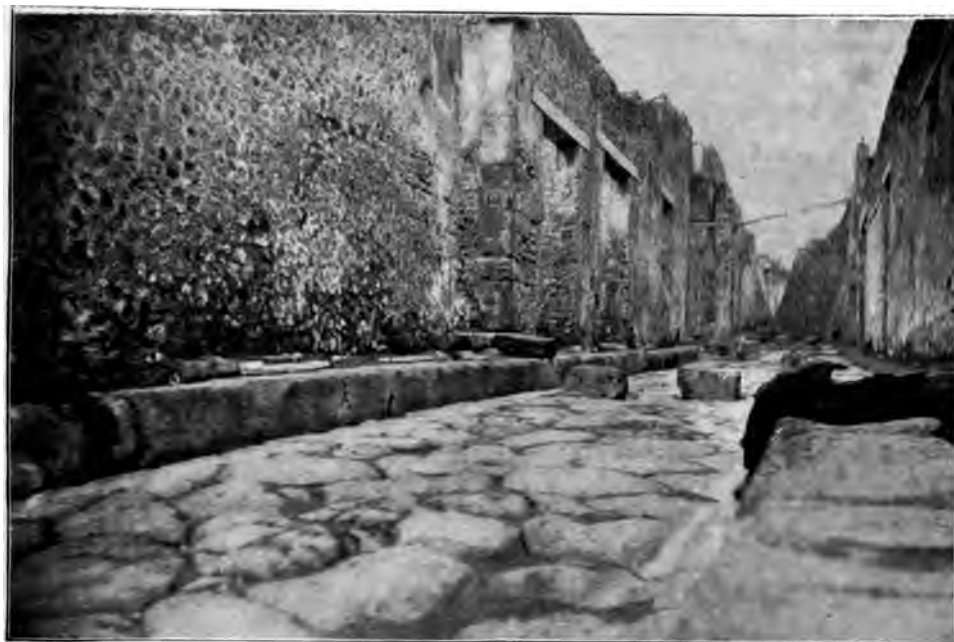
LEAD PIPE LAID IN THE STREETS OF POMPEII ON THE SIDEWALKS. 2
